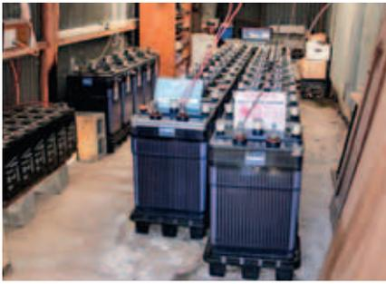
to power each of the three strings of batteries; each panel has its own isolating switch. Due to the size of the battery banks, we have never used a regulator and will only reduce the charge manually (turn off a number of panels per set) if we are away for extended periods.
